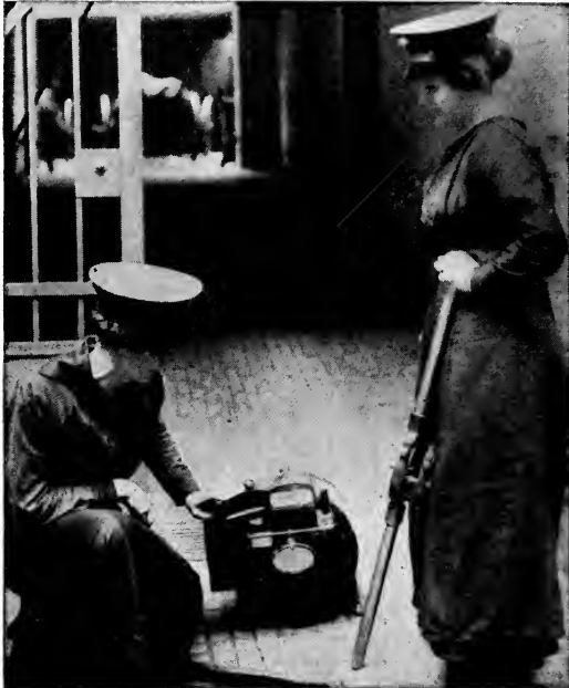
Reading the Gas Meter.
